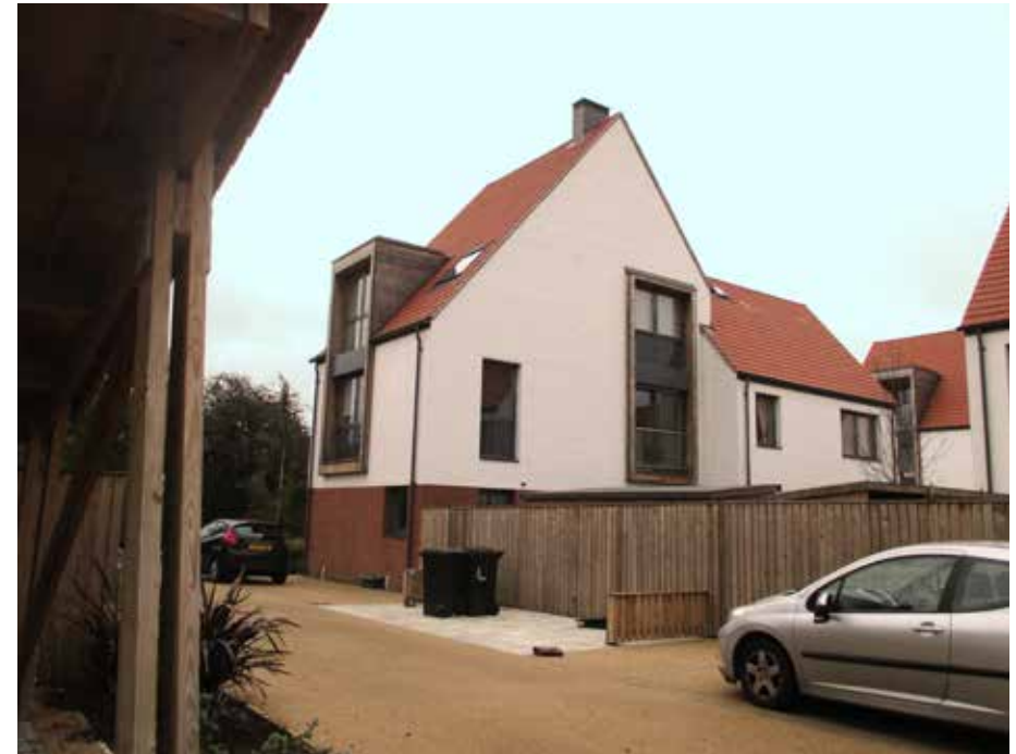
Figure 7 Bin collection area at Derwenthorpe, York. Collection areas to the sides of houses, away from people's windows and doors, are marked out with paving slabs and low fences
