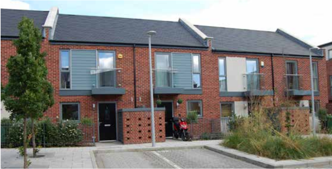
Figure 3 Ventilated robust structures at Centenary Quays, Southampton
