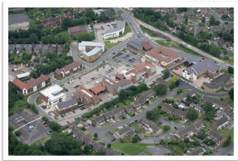
Figure 13 - Lintot Square from the air
