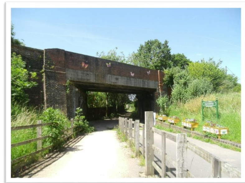
Figure 9 – Looking north up the Downs Link adjacent to Lintot Square.
